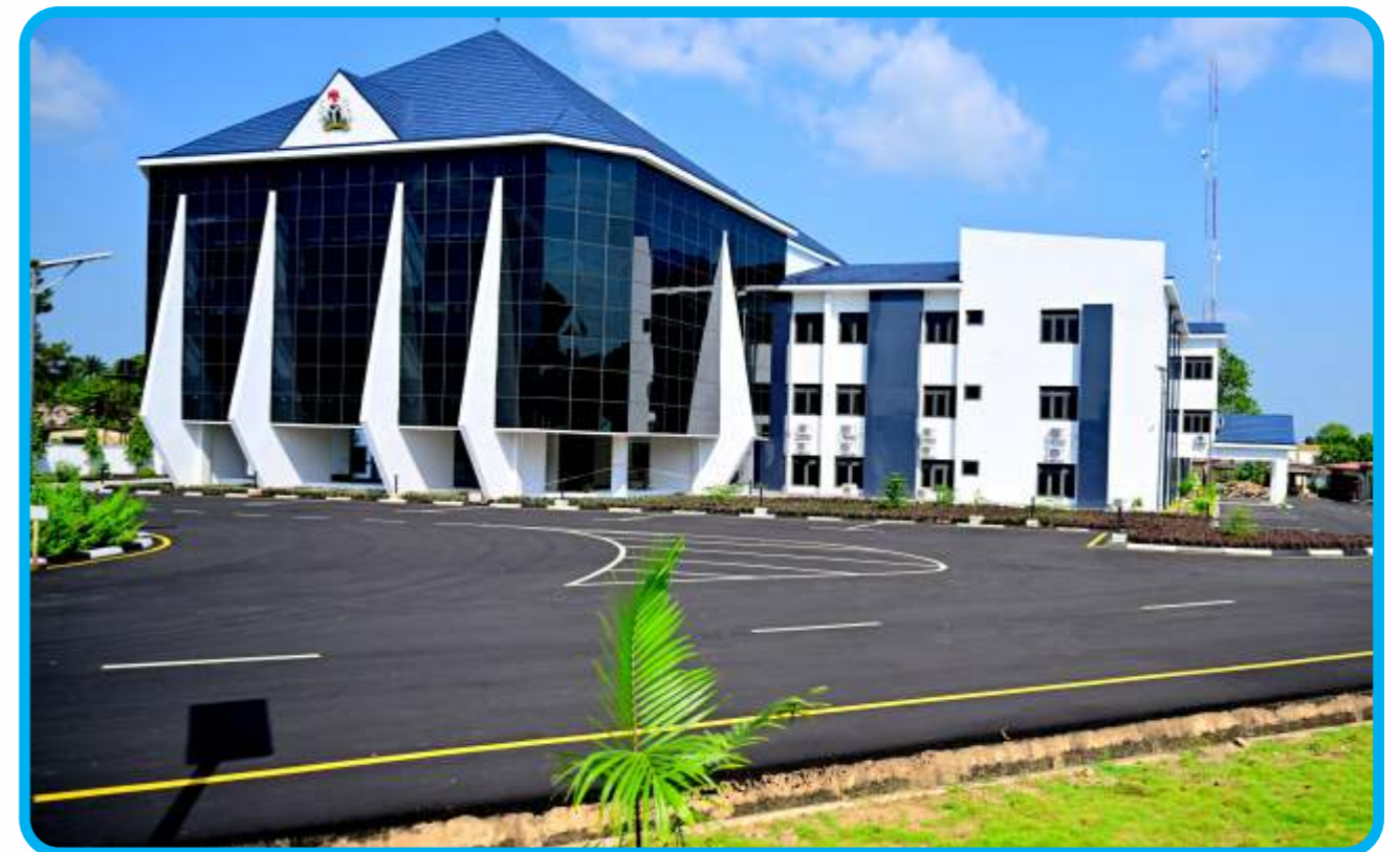
NEW LOOK GOVERNOR'S OFFICE, (GLASS HOUSE) CALABAR COMPLETED BY GOV. OTU
