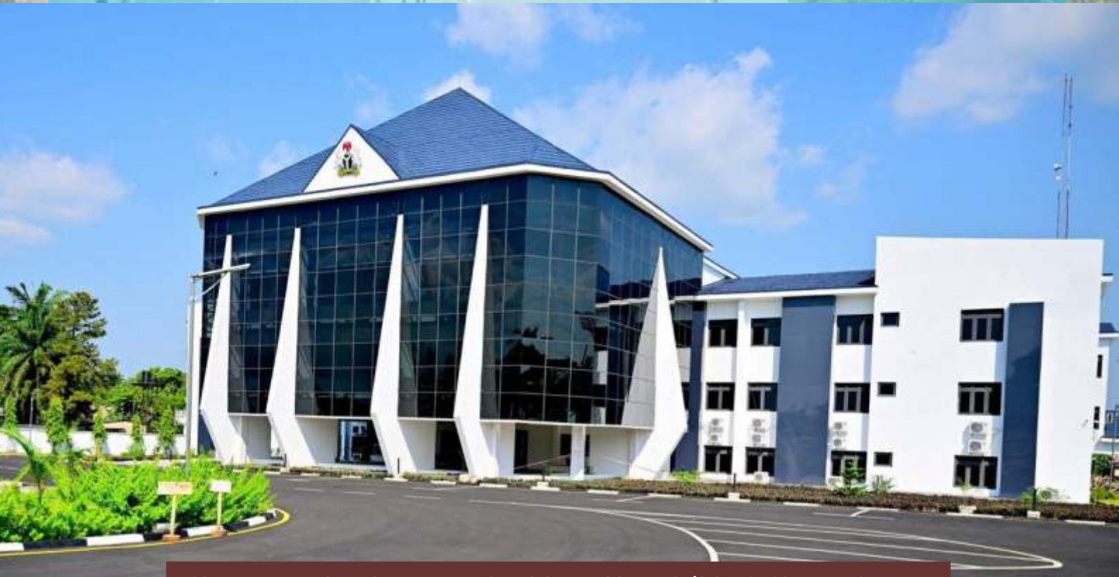
COMPLETED RENOVATION AND FURNISHING OF THE GOVERNOR'S OFFICE COMPLEX, CALABAR
